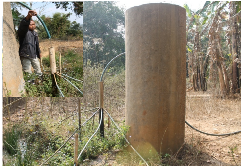
Figure 4.15 Adapting to available resources: Seen in the picture is a innovative method of storing water, sourced from a stream located at a higher altitude, in a 'Hume-pipe' (meant for use in pipe-culverts during road construction) and distribution to households in a village called Silaguri in Karbi Anglong.
