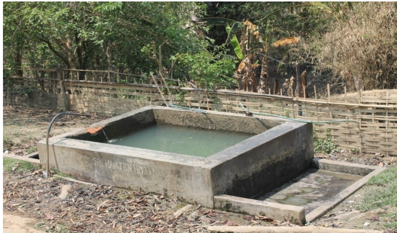
Figure 4.14 Water Supply arrangement provided by PHE at Hojai Khasiba Village, Dima Hasao
