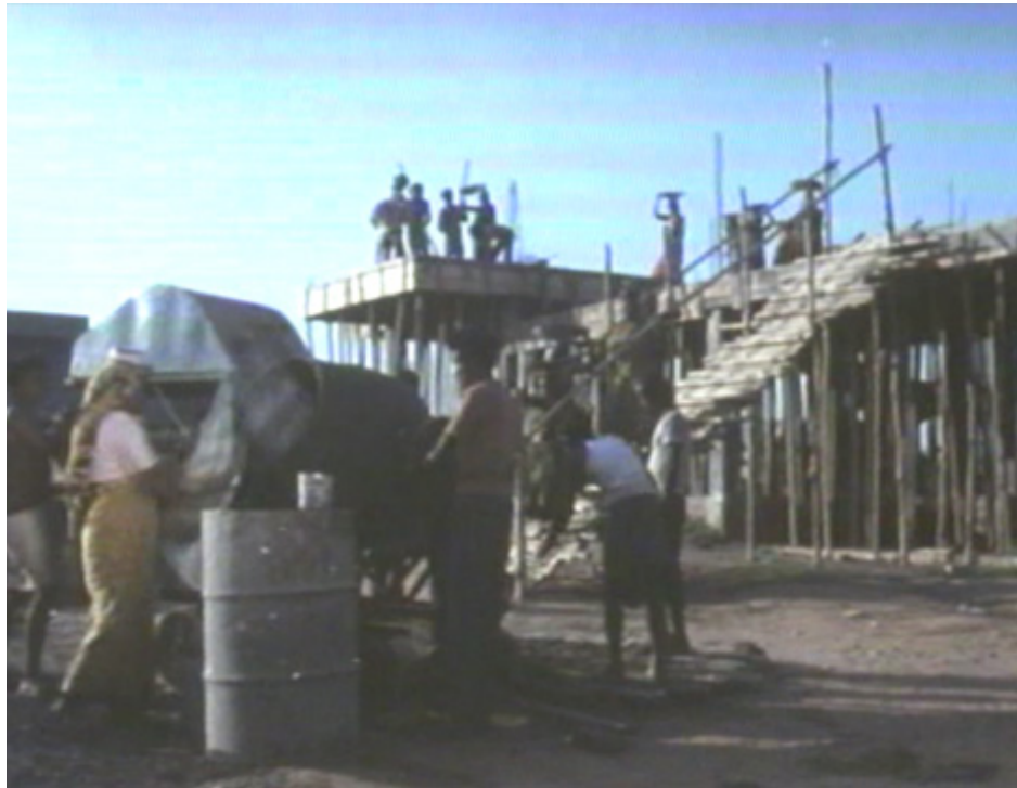
Figure 21: The house-construction site in Sarothi
