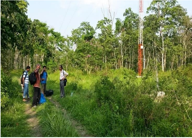
Photo 3.5: Installation of sensors on the tower during 2014
