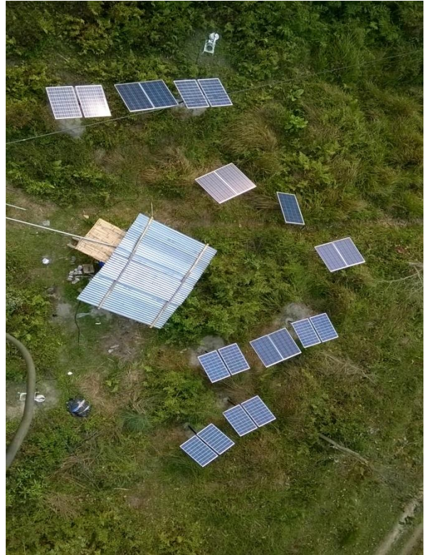
Photo 3.2: Solar panels around the tower
