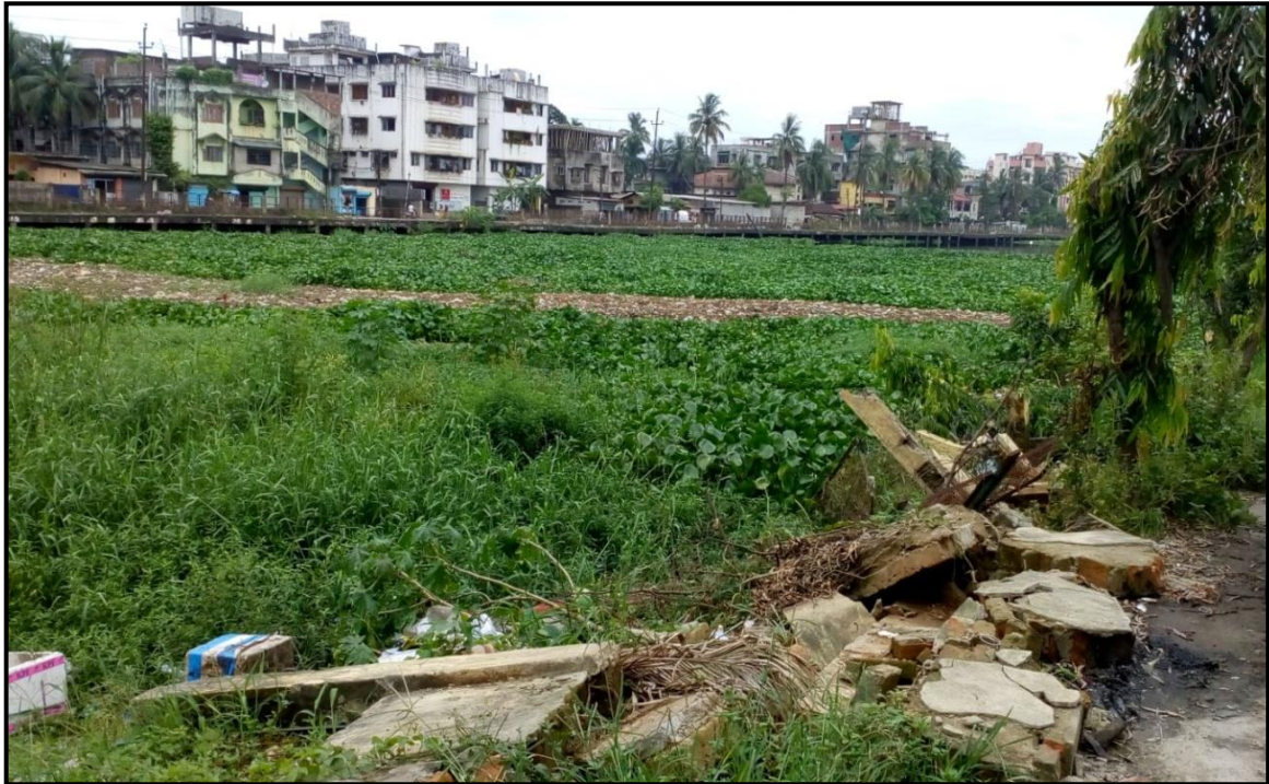
Figure 5.10: Rubble from construction activities
