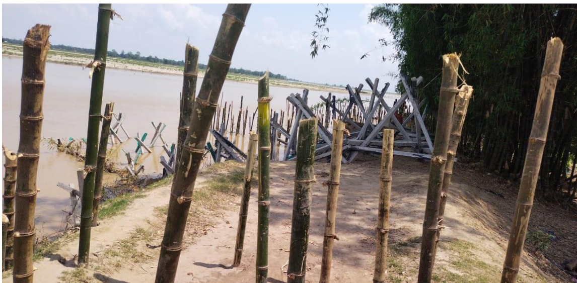
Image 5.2 Bamboos and porcupines are used together by the villagers to break the water currents of the river and avert its intrusions towards the village. Photo taken on 18 th December, 2021.
