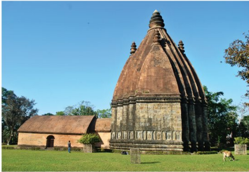
Figure (xi) : The complete structure of the Gaurīsāgar Devī Doul, Sivasagar district The Maṇḍapa ( on the left ) followed by the Antarāla and then the Garbhagrha enclosed by the Pañcaratha Bāda structure topped by the Śikhara of the type known as Kardaisiriyā or Jikāsiriyā ( on the right )
