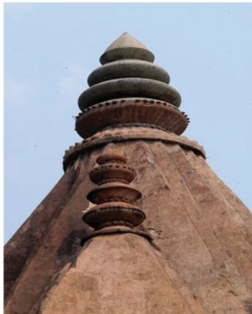
Figure (xii) : The structure of the finial or apex of the Śikhara of Gaurīsāgar Devī Doul
