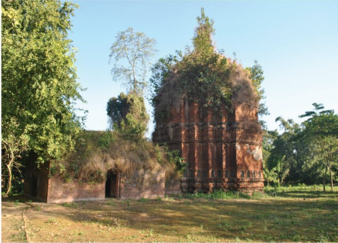
Figure (xviii) : The Jagaddhātrī Doul, Kalugaon, Sivasagar district before its restoration
