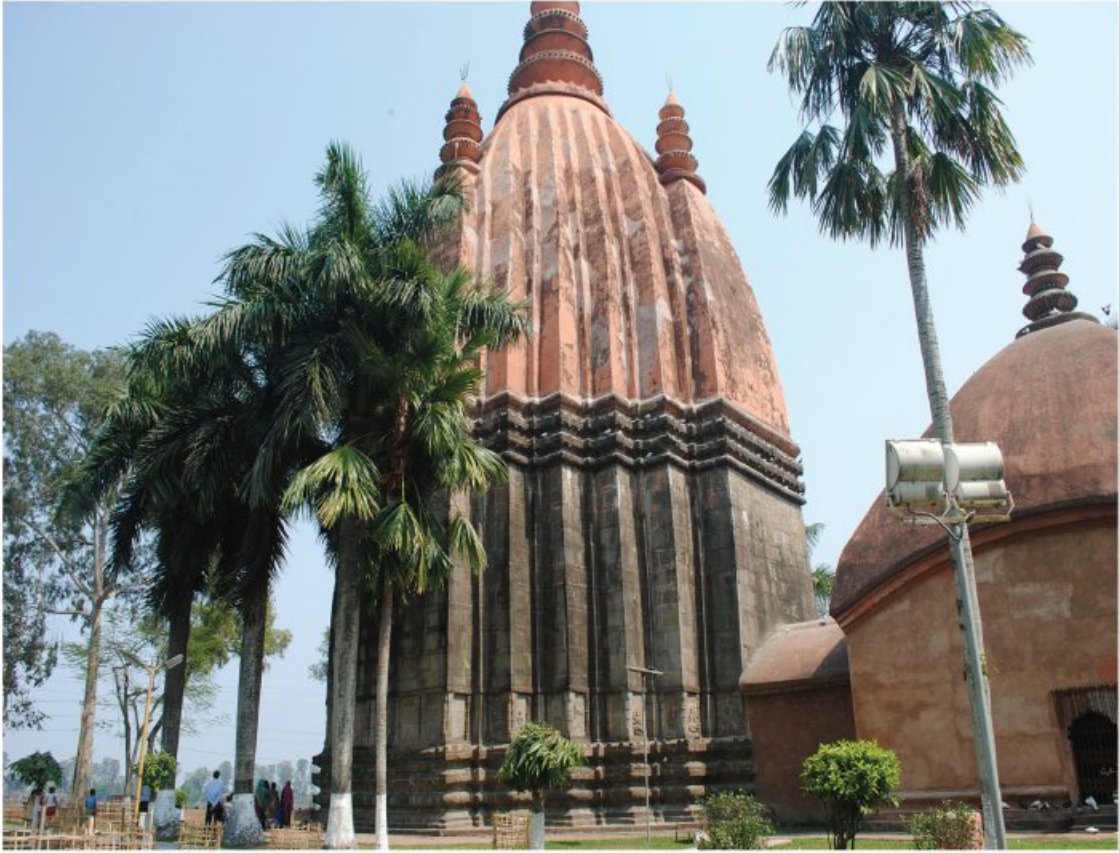
Figure (xv) : The Bar Pukhuṛī Śiva Douḷ, Sivasagar district The Cou Cāli structure ( on the extreme right), leading to the Antārala having a Do Cāla roof. The Antārala leads to the Garbhagrha enclosed by the Bāda topped by the curvilinear composite Śikhara
