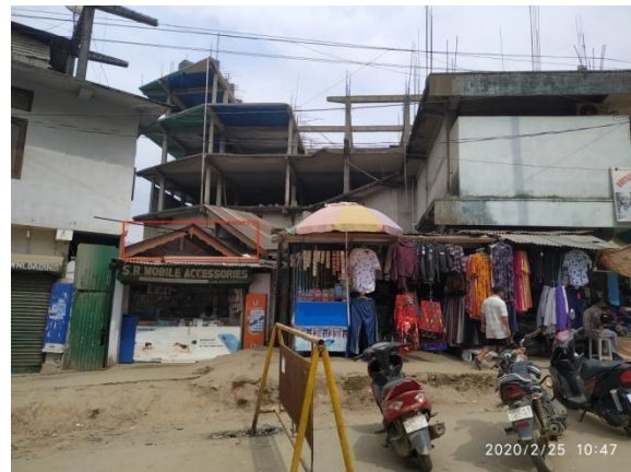
Figure 5.4. Government Quarter Encroachment 4
