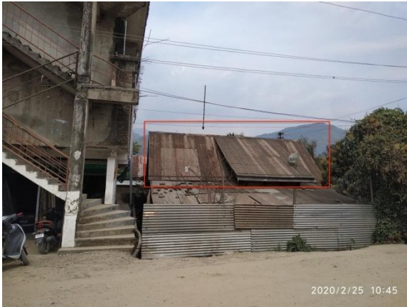
Figure 5.1. Government Quarter Encroachment 1
