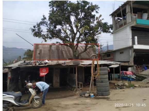
Figure 5.2. Government Quarter Encroachment 2
