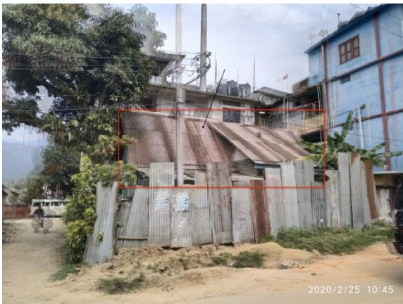
Figure 5.3. Government Quarter Encroachment 3
