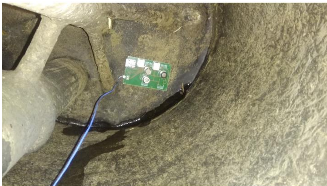
Fig 4.4 (a): Installing the circuit inside the digester
