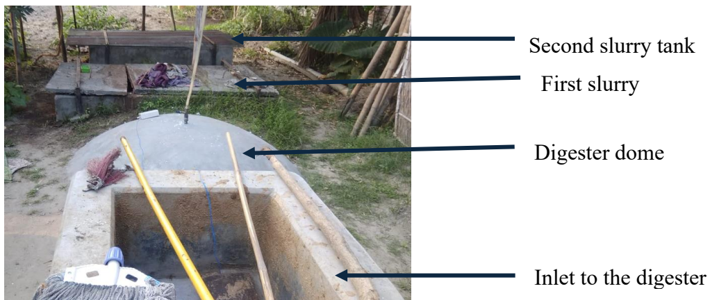
Fig 4.7 a: 2 cubic meters Deenbandhu biogas system
