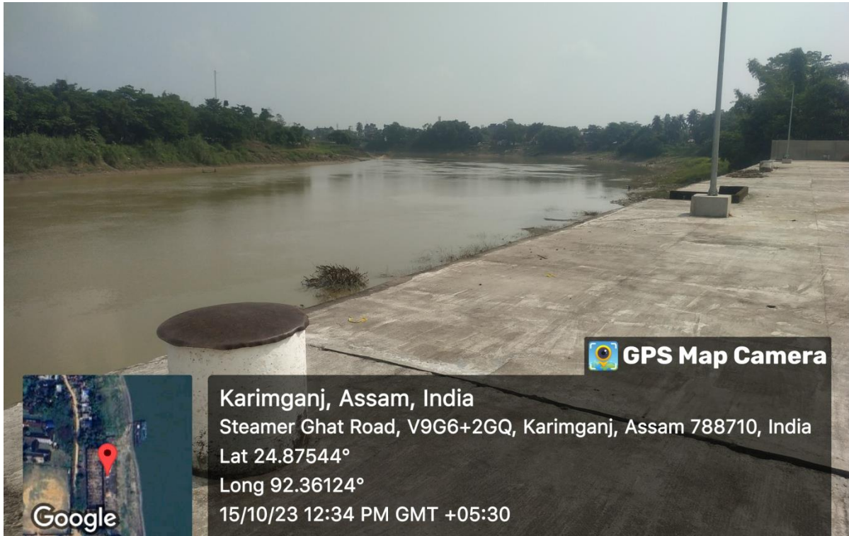
Plate 11: RCC Jetty at Karimganj port
