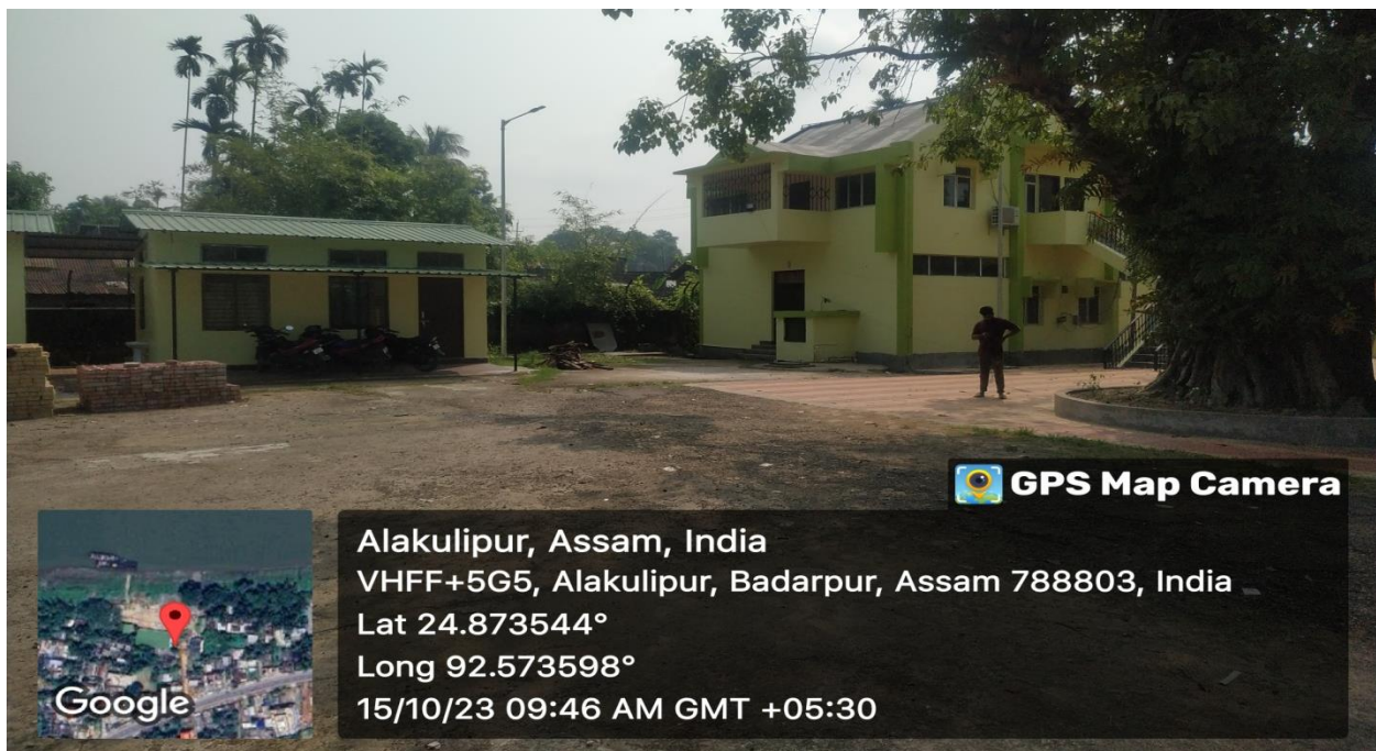
Plate 16: IWAI Terminal Office at Badarpur port
