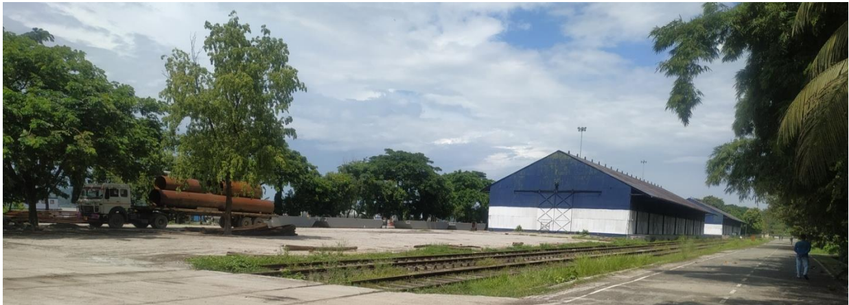
Plate 5: Sheds and railway track at Pandu Port
