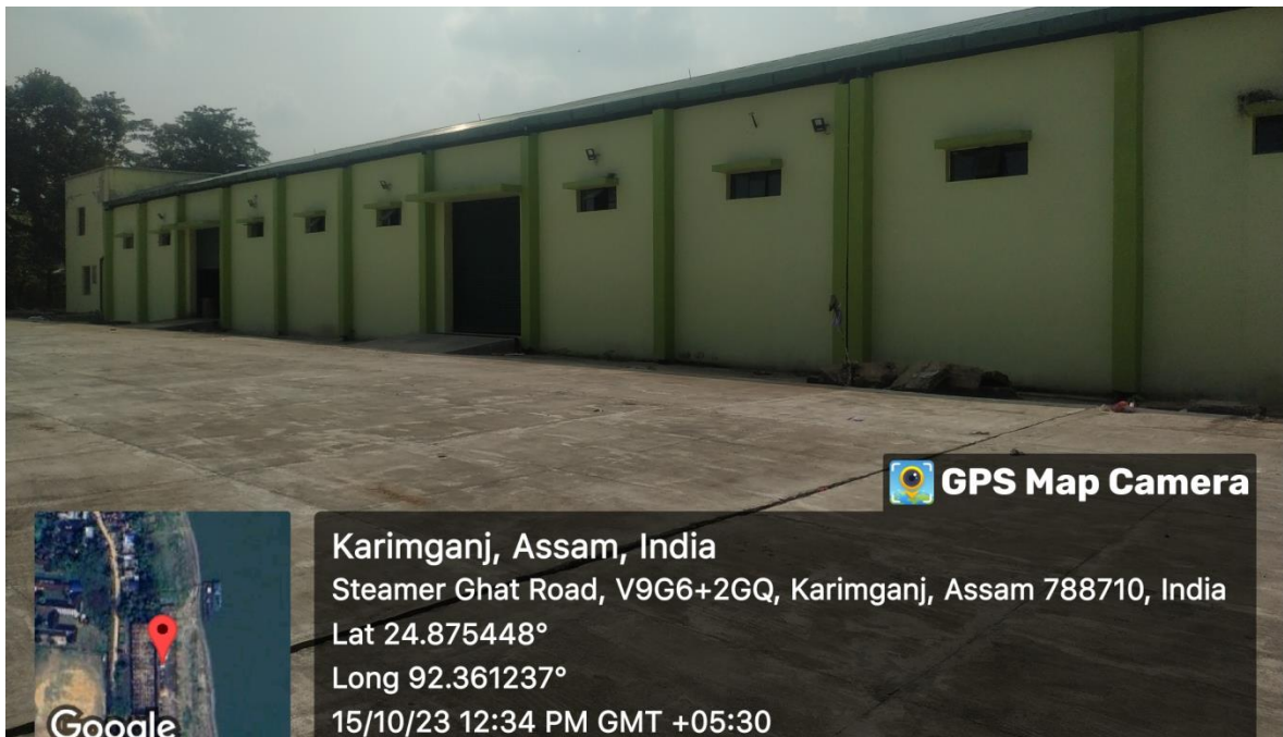
Plate 12: Covered Shed at Karimganj port
