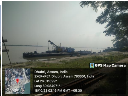
Plate 4: Floating Terminal at Dhubri Port
