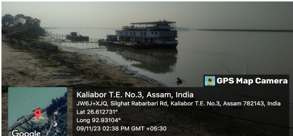
Plate 9: Floating Terminal at Silghat port
