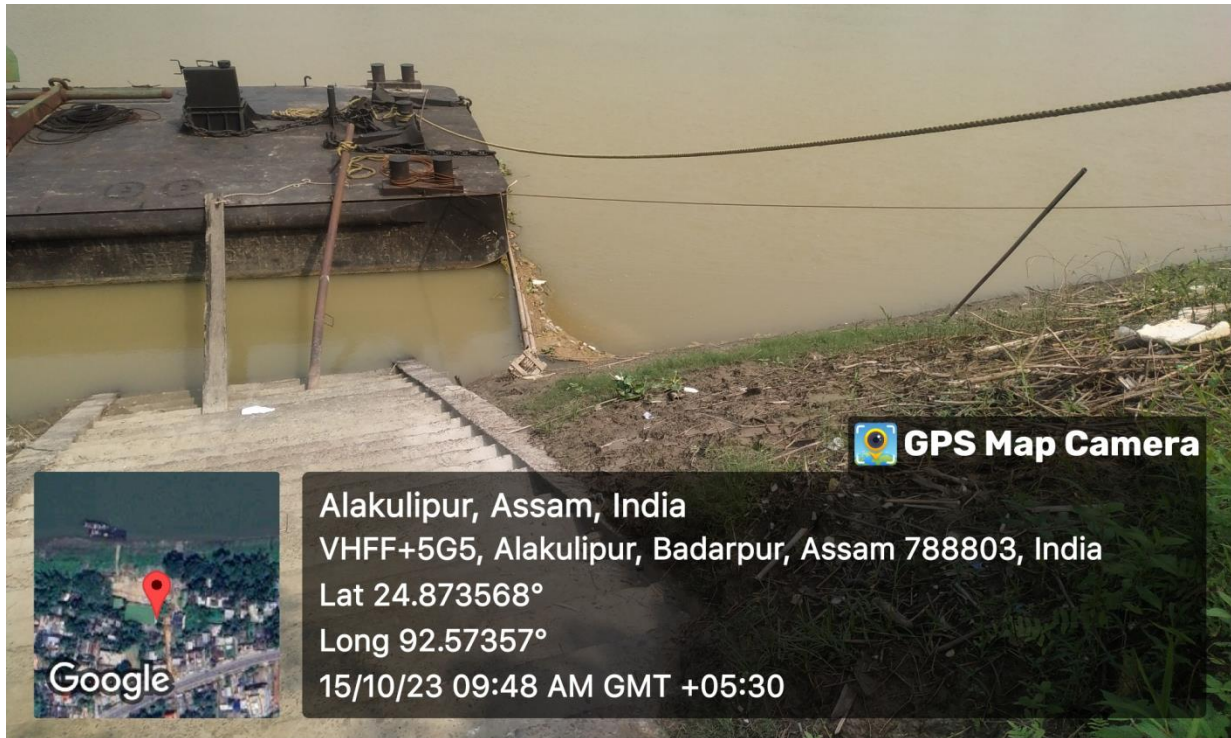
Plate 15: RCC Jetty at Badarpur port
