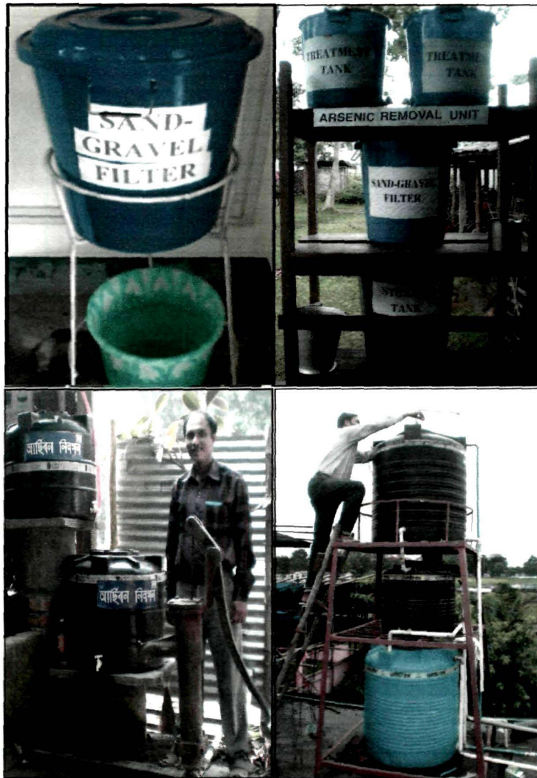
Figure 2.5. Arsenic removal systems of different capacities (a) 10 L; (b) 25 L; (c) 200 L; (d) 500 L.
