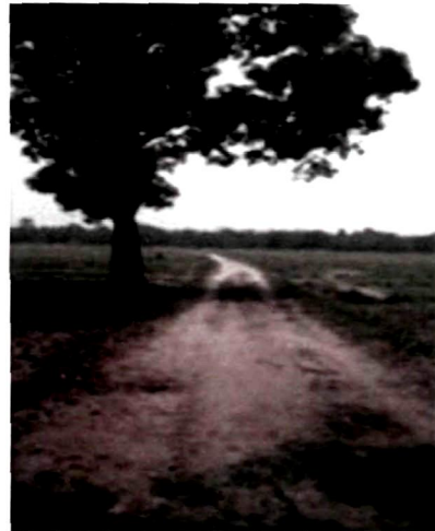
28. A kuchcha constructed by the villagers in Sopaloga under the JFM Scheme
