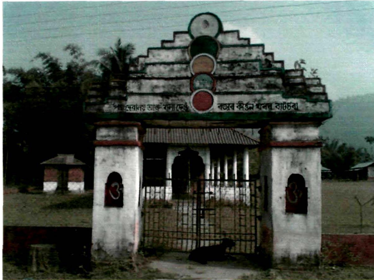
Photo 23: Entrance of the Kirtan-Ghar of Khola Deo- Raja
