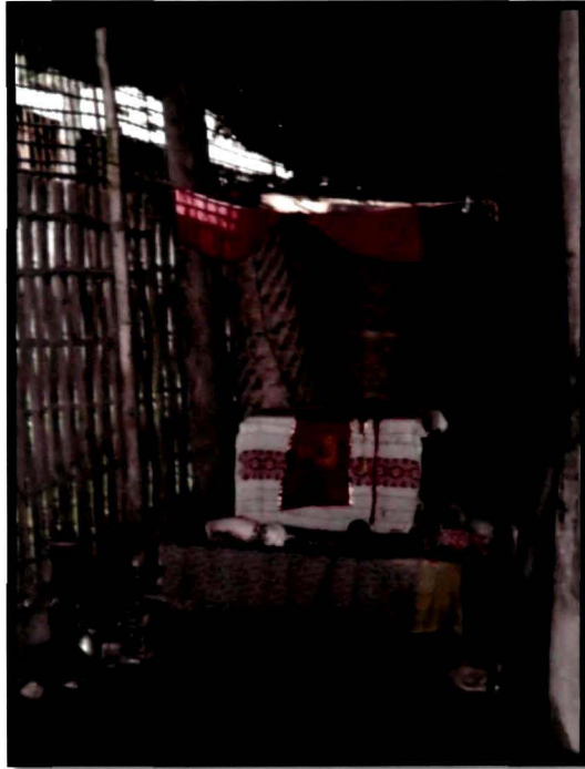
Figure: 30 - The dilapidated state of the nāmghar at Letugram Sattra.
