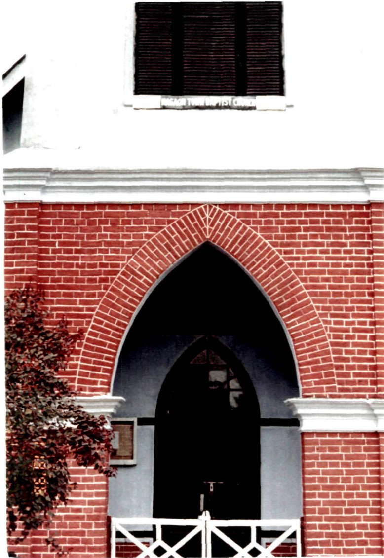
Brickwork in English bond with an arched lintel at the entrance to the Nagaon Town Baptist Church, Nagaon, Assam
